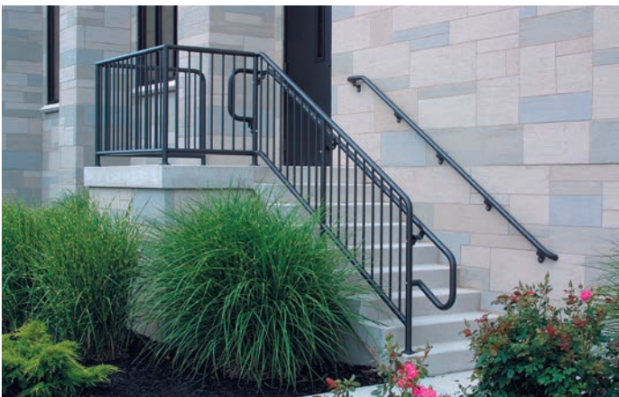
Superior Series 500 Non-Welded Aluminum Pipe Railing (hand rail at steps). Superior Series 550 Non-Welded Aluminum Pipe Picket Railing (at steps and landing).
